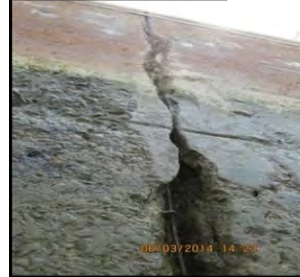
Monolith Joint Deterioration
